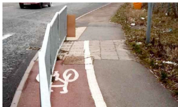
Fig 1. Example of conflict between design standards
